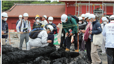
Inspection of the damage
