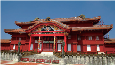
The Main Hall will be restored using local timber
